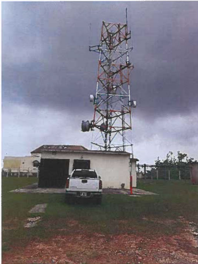
Guam Police Department- Maintenance Building
